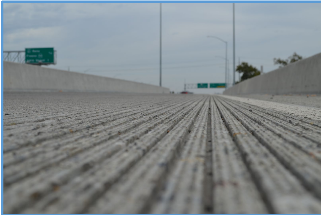
FIGURE 6 Top: Red lines show easily identifiable and loud, transversely tined surface texture pattern on Google Street View map, Bottom: Close-up of quiet longitudinal Groove-and-Grind rigid pavement texture used both on and off Caltrans structures.
